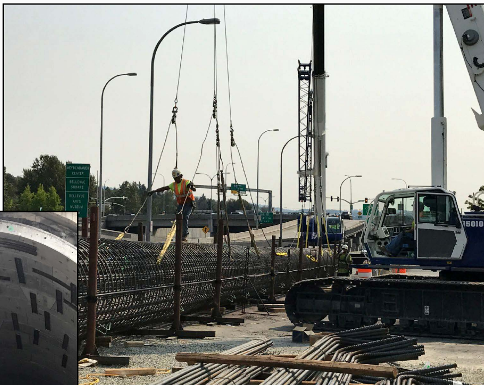
Stacey & Witbeck E335 project. Mark Mills and Todd Anderson - Crane Operators
