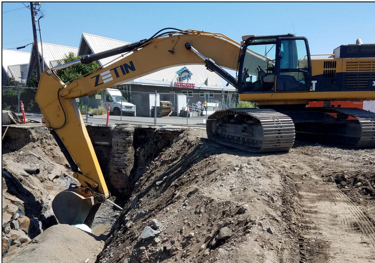
Zetin Construction CSO Tank Spokane WA - Jeff Berger
