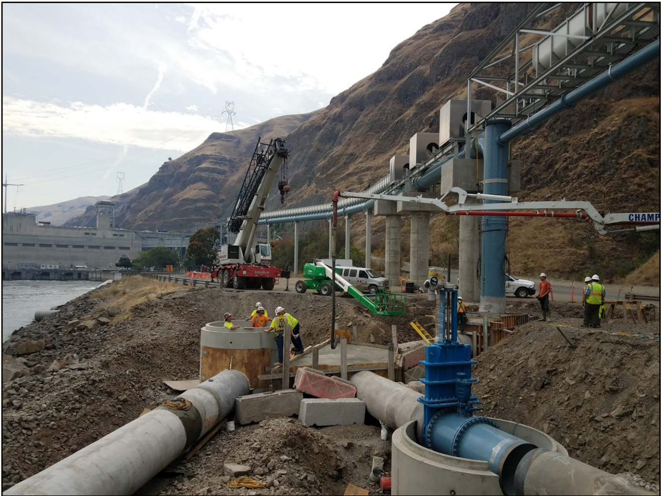
Garco Con. Lower Granite Dam, New Fish ladder.
