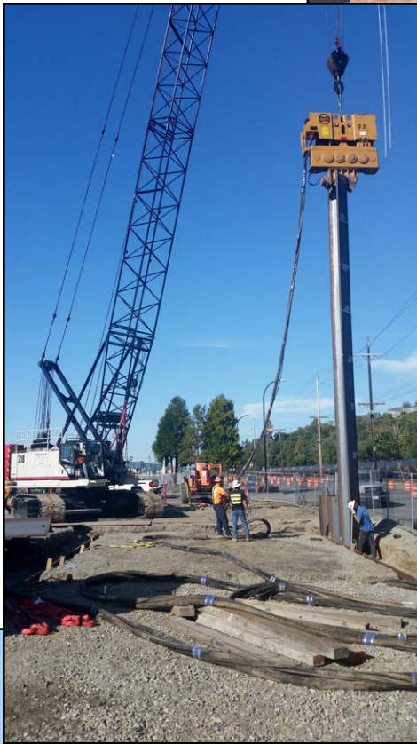
ICI New 218 Linkbelt Crane driving Sheet pile on the Grand Avenue Park Pedestrian Bridge over Marine View Dr, Port of Everett, Operator Michael Schumacher.
