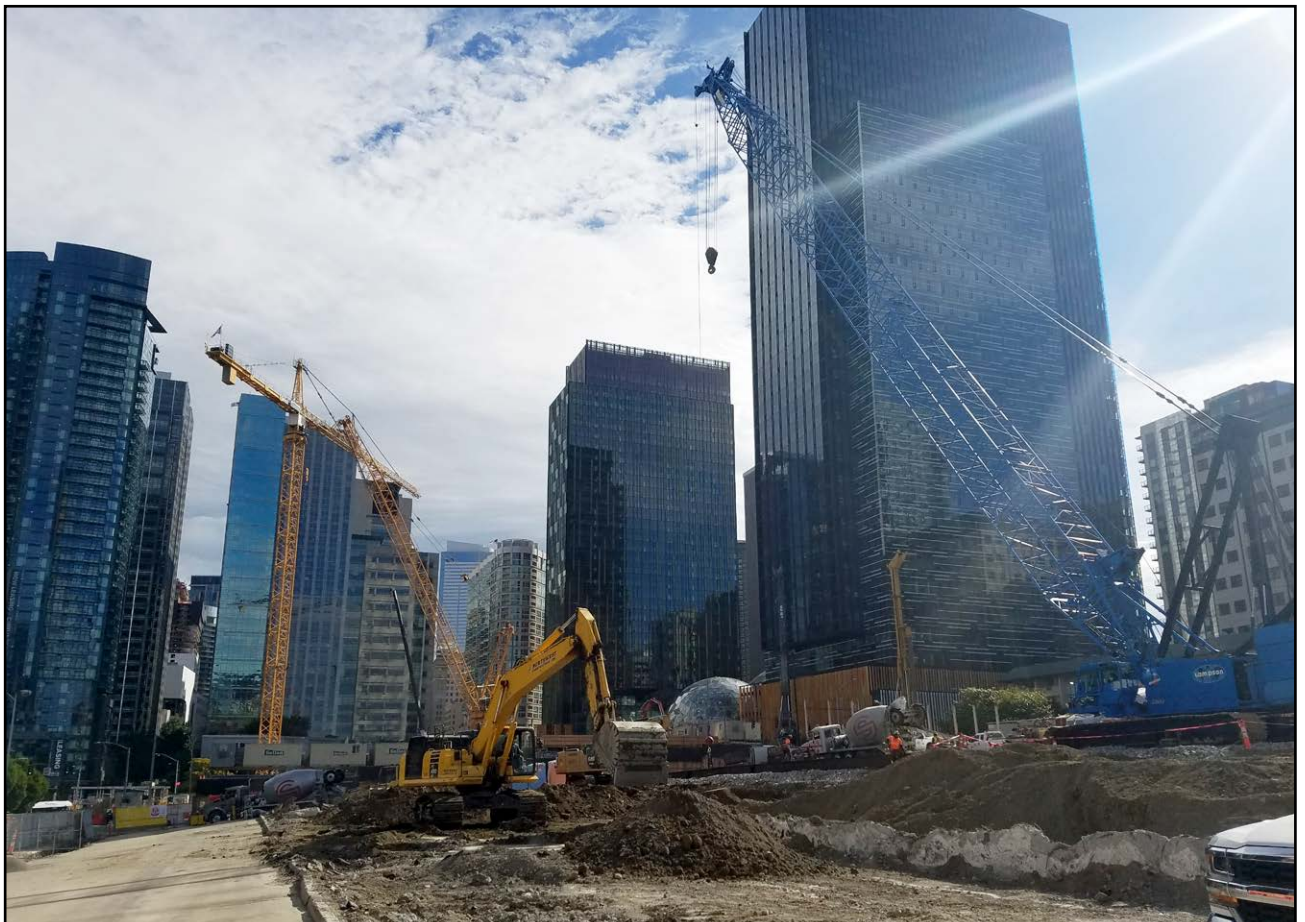
GLY breaking ground on Amazon's block 21 project in Seattle
